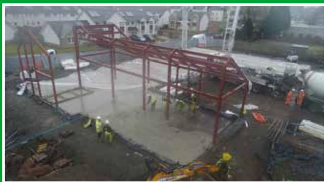
This picture, captured by a drone from McNiven Construction, shows the structural steelwork in place for the new £2.7m Doune Health Centre. Underground drainage has been completed and the concrete floor slab laid. Work is now under way on the building itself, which is due to open later this year.
